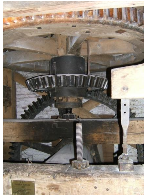
The mill wheel at Mapledurham, Oxfordshire, drove the cogs turning the grindstones, © Hilary L. Turner
