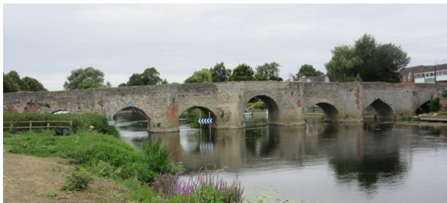
The upstream side of the bridge at Bidford on Avon; built originally in the fifteenth century, the semi-circular arches mark repairs carried out after deliberate destruction in the early 1650s. © Hilary L. Turner
